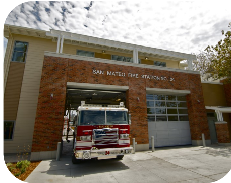
San Mateo Station 24—319 S. Humboldt St. Engine 24—3 personnel
