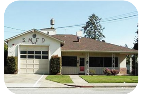
San Mateo Station 25—545 Barneson Ave. Engine 25—3 personnel
